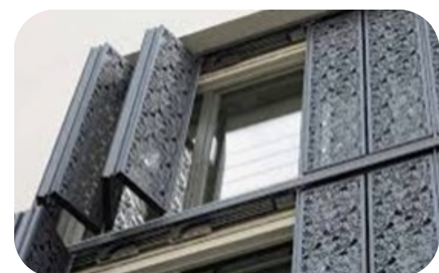
V1 - VOLET PLIANT-COULISSANT Aluminium-Acier- ACM- NidA-Fibre-ciment
